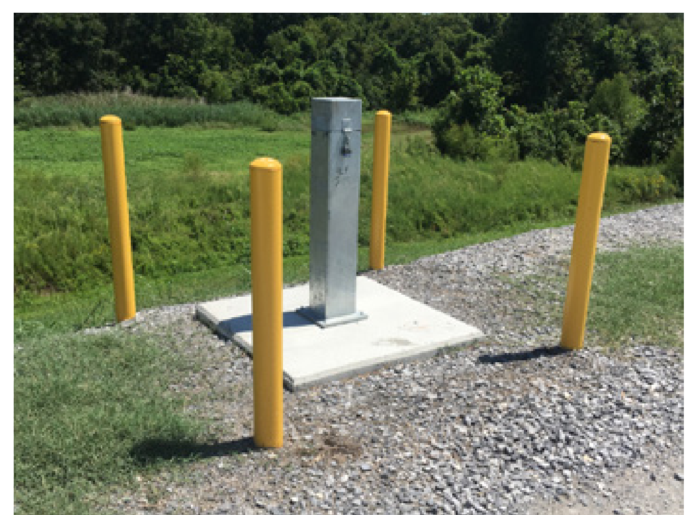
Groundwater monitoring well
