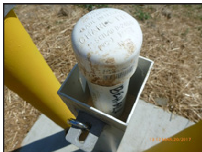
Surface protection for top of well
