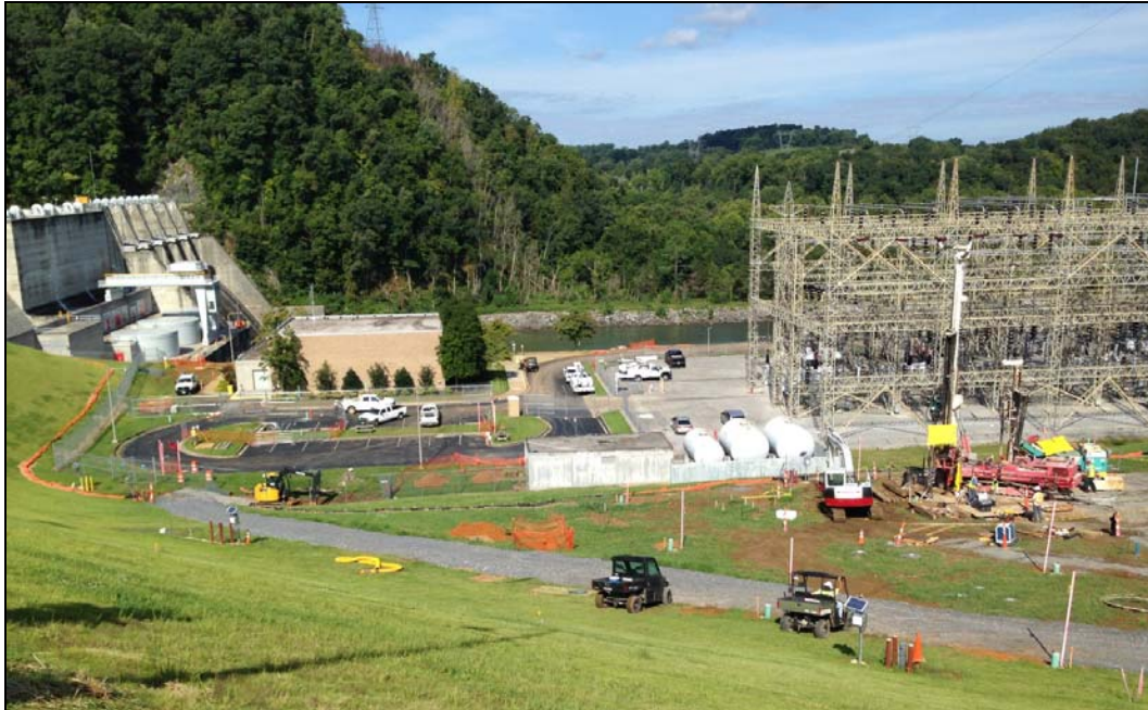
Photo 3-10: Ongoing Construction Activities at Boone Dam
