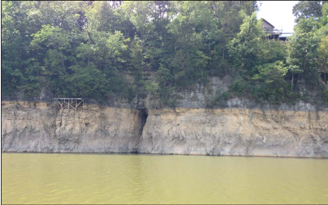
Photo 3-2: Exposed Cave Opening below the Typical Summer Pool Level
